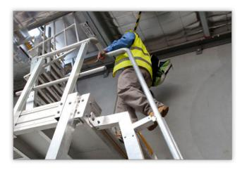
Two factors make step-type ladders safer than rung-type ladders: stability and balance.
